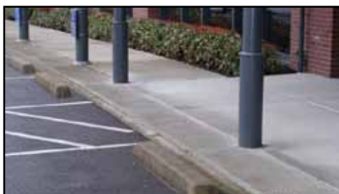
In the photograph on the left, the tire bumpers protect structural supports to an awning. In the photograph on the right, the tire bumper may be able to be removed.
