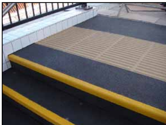
If stairs in your facility don't have good slip resistant properties, it may be possible to retrofit the stairs to achieve significant improvements. "SlipGrip Stair Tread Covers" is one example of a product that provides a rough surface on each stair tread to give people more traction.
