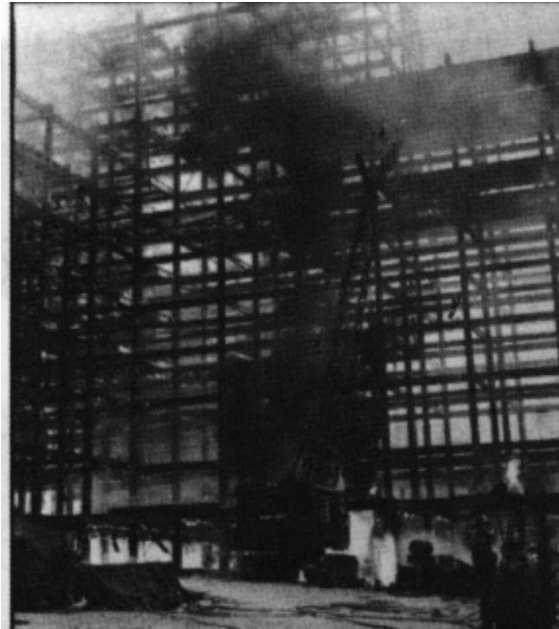
Figure 4. Firefighters preparing to extinguish a blaze that began at the foundation area of this building project. Storage areas should be located far enough away to avert a possible fire.
