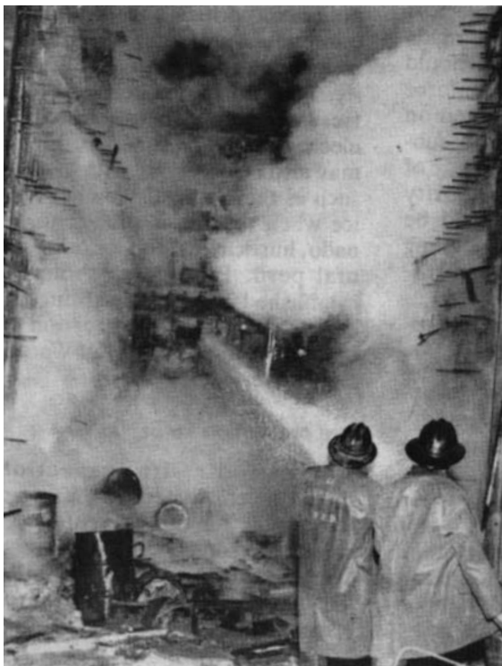
Figure 1. Good housekeeping could probably have averted this building construction fire.
