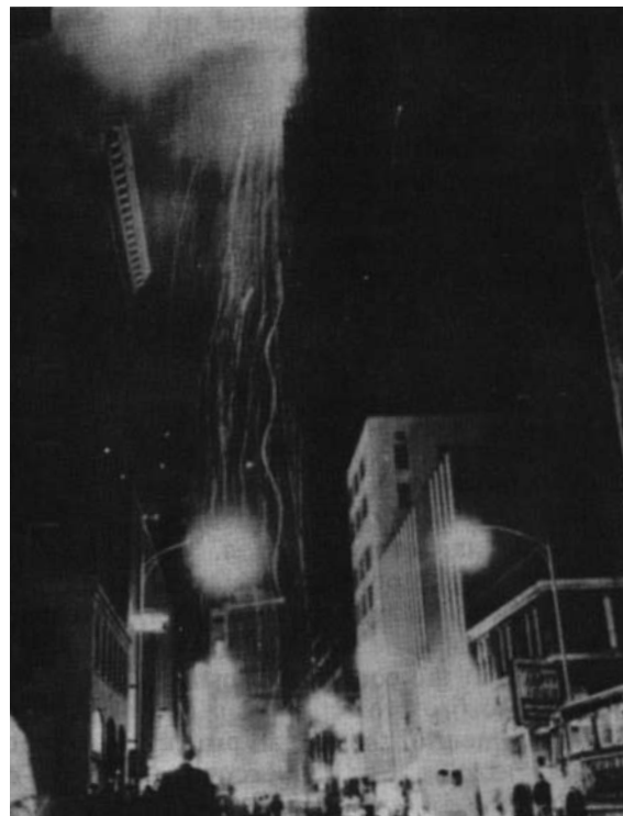
Figure 2. Flaming debris showering down from atop this blazing 34-story building under construction. Fortunately, there were no serious injuries.
