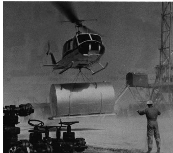
**Figure 5** shows a signalman at a worksite who is directing the operation of a helicopter carrying a portable field storage tank on skids.
