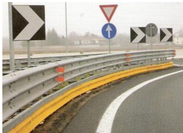
Image 2: Example of modified guardrails
