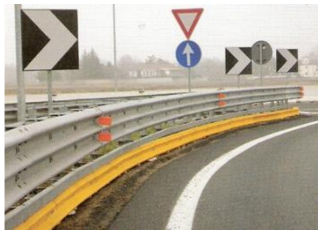
Image 2: Example of modified guardrails
