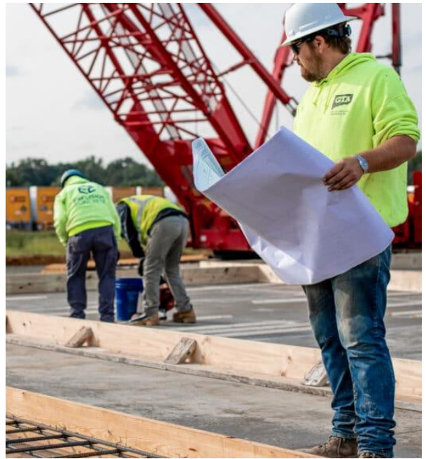
Figure 1. Outdoor workers are often exposed to heat-related hazards like sun exposure, high temperatures and limited access to shade and water.
