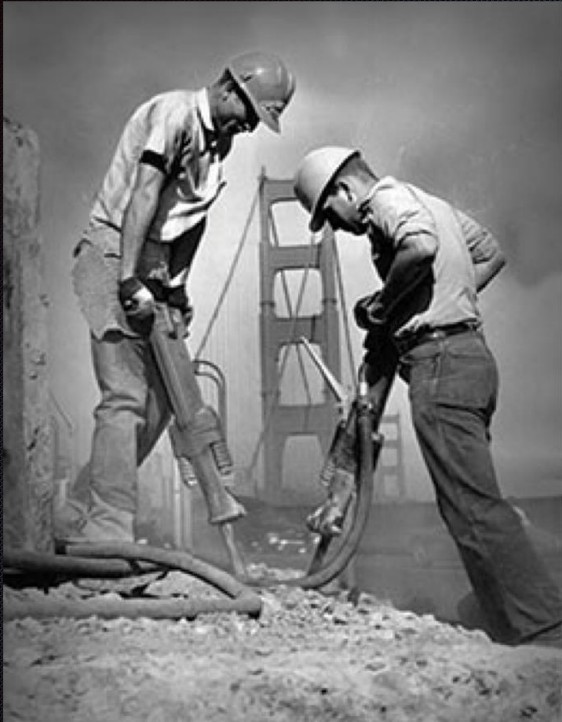
Golden Gate Bridge
